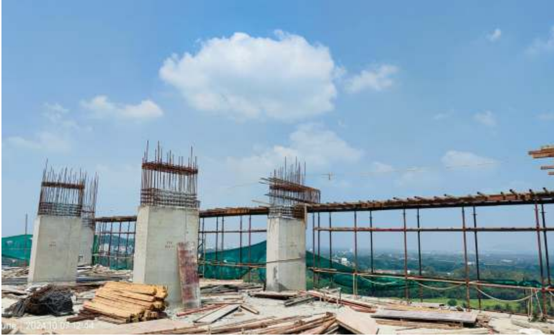
Terrace slab RCC Work in progress.
