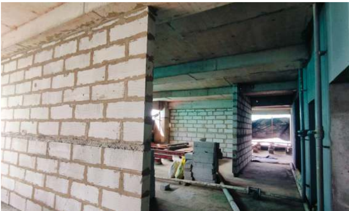
13 th floor internal Blockwork in progress.
